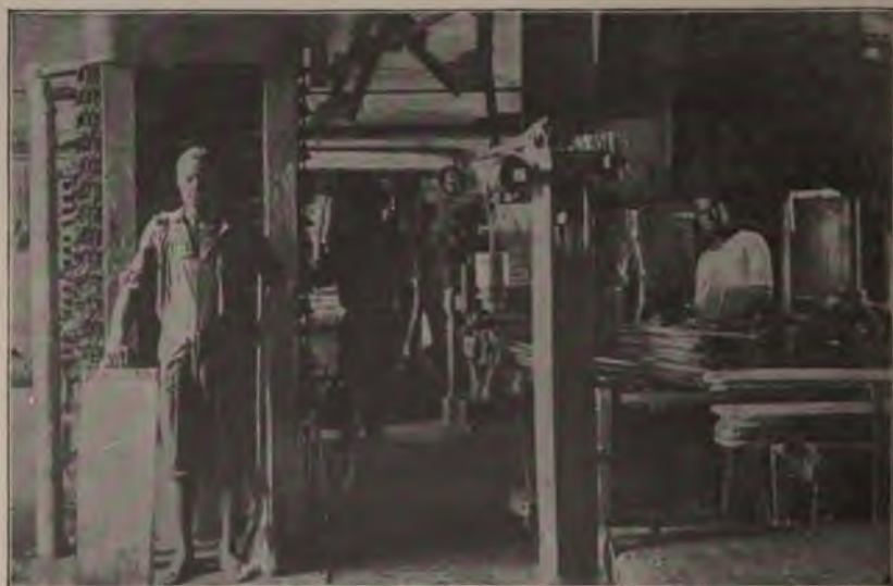
FIG. 57.—REMOVING THE OIL CAKES FROM A COTTONSEED PRESS.—(Courtesy of David Wesson.)
